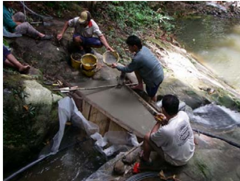
Community project - Construction of water dam for gravity feed water supply
