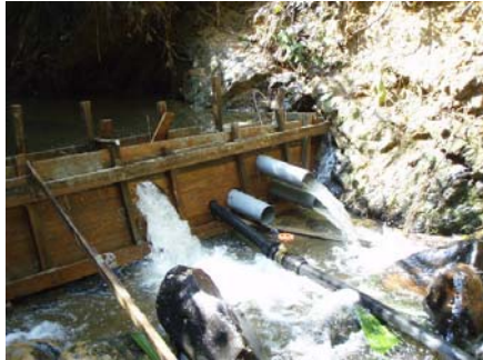
Community project - Water dam for gravity feed water supply
